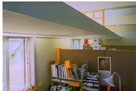
South-facing windows combined with light shelves provide daylighting for first-floor work spaces. The light shelves bounce light through interior clerestory glazing into north rooms more than 30 feet away.
