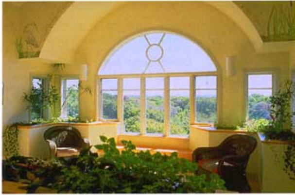
Large south-facing windows in the second story welcoming area provide direct solar gain and an expansive view of the Atlantic Ocean.
